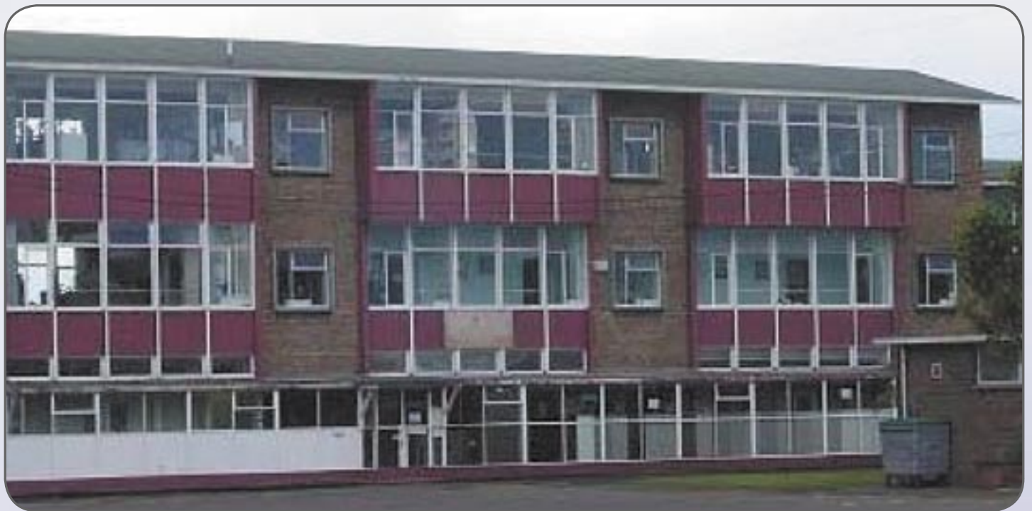
Typical local authority SCOLA building with single glazed steel windows - benefits greatly from MISO 2000
